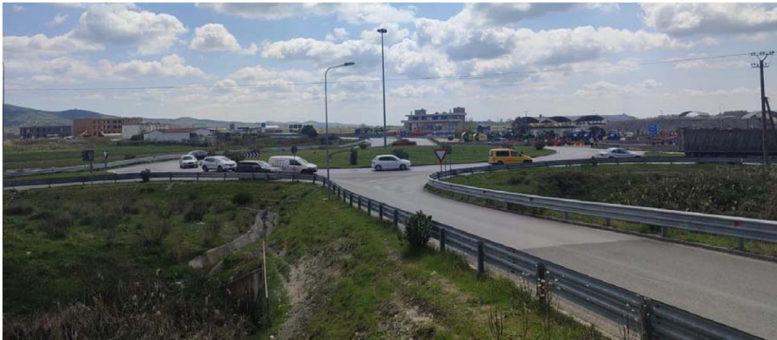
Photos from the field, road condition
