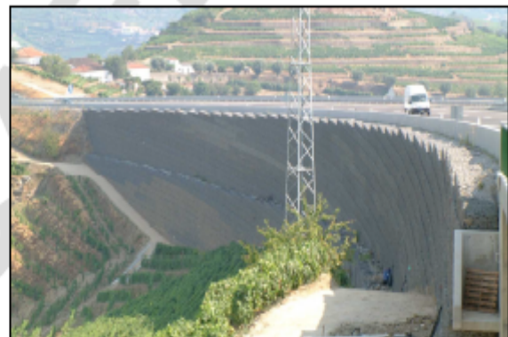
Terramesh installation
